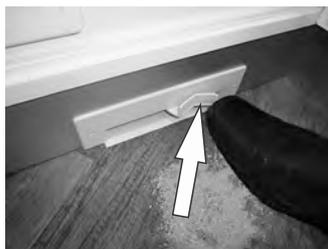
3. Any dirt/debri close to the inlet area will then be sucked into the vacuum unit.
