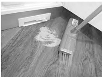
2. Using your toe, gently push the lever of the dustpan inlet point inwards. This will automatically activate the vacuum unit.
