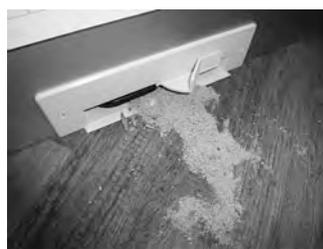
4. Using your toe, gently push the lever of the dustpan inlet point outwards. This will automatically turn off the vacuum unit.
